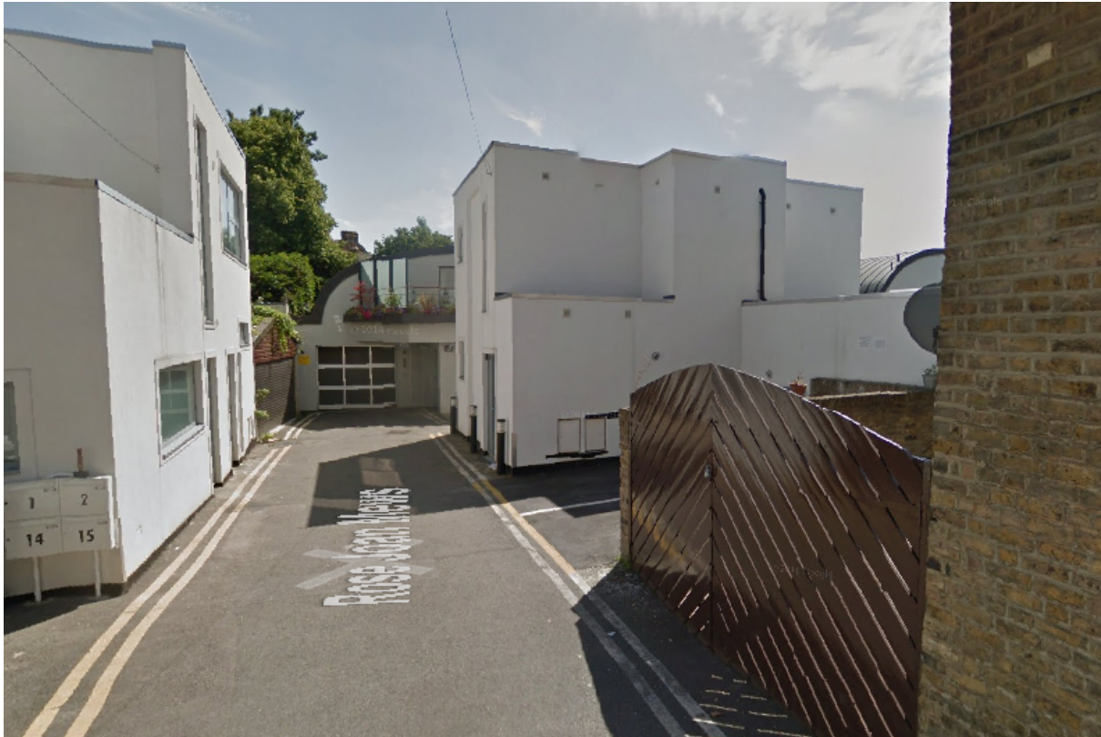
Photo 1 – View of the rear elevation of application site
