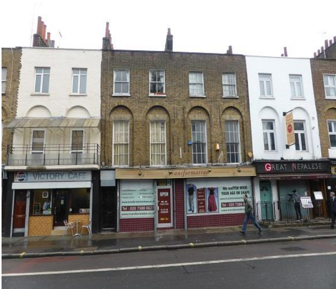
Photograph 1 - Showing the front elevation of Eversholt Street London NW1 1DA
