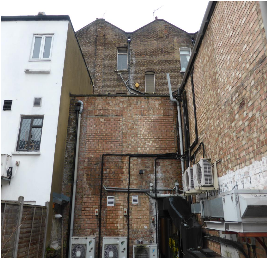
Photograph 2- Showing the rear elevation of Eversholt Street London NW1 1DA
