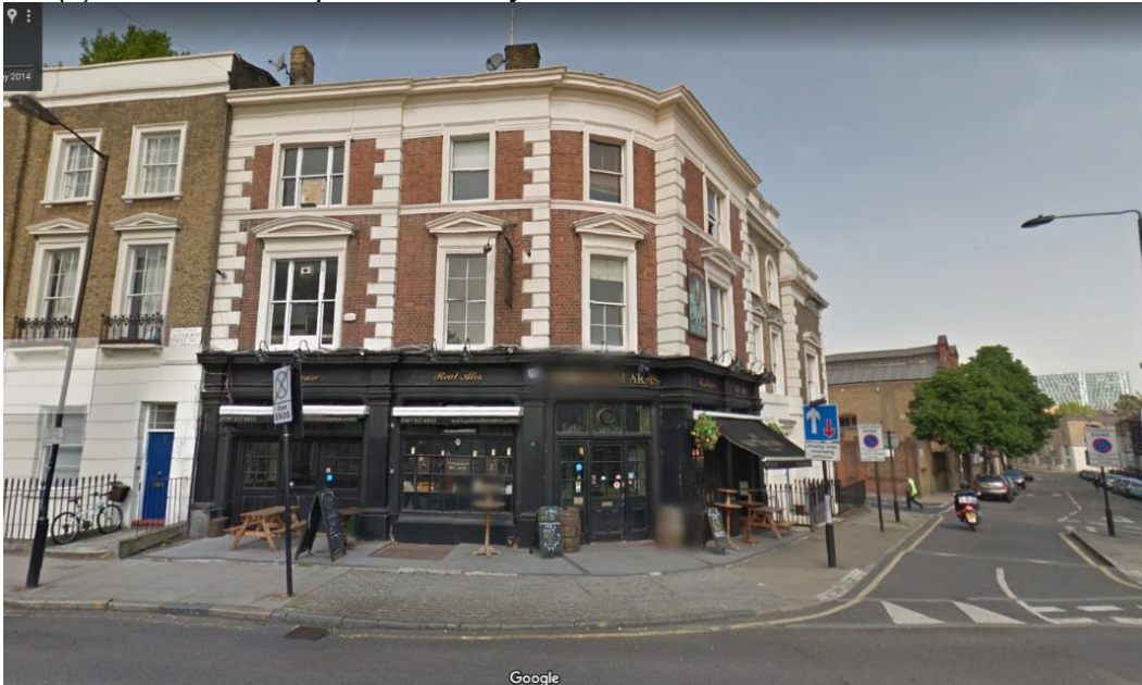
(4) Public house closes in preparation for works to commence (July 2014)
