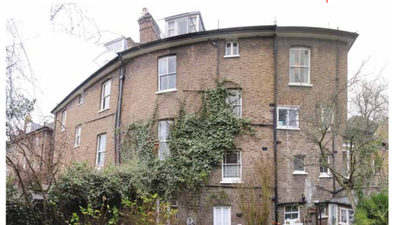
Fig 3.D Rear Elevation of number 22 South Hill Park Gardens and adjacent properties
