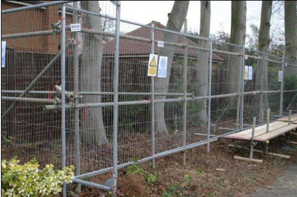
Figure 2: An example of ‘floating’ ground protection
