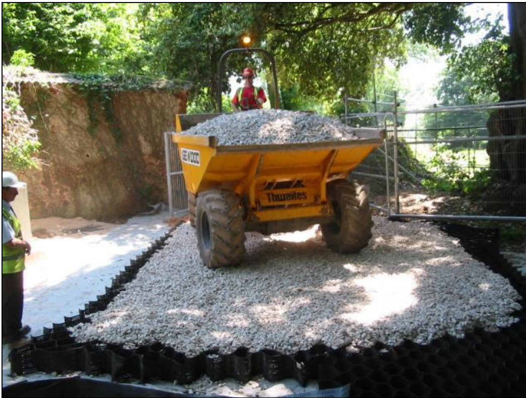
Figure 5: An example of a no-dig driveway under construction
