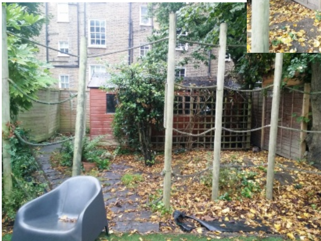
Rear of garden to 187 - site of new garden building
