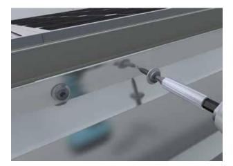
The individual wind deflectors must be connected at the overlap positions using self-cutting thin sheet screws fitting in the pre-drilled holes. The minimum overlap of the sheets is 90 mm. The wind deflectors must be aligned such that the thin sheet screws in the area behind the wind guide have a distance of at least 20 mm to the edge.
