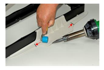
Hand welding of the flaps along the length of 280 mm between the arrow marks on the Sika SolarClick. The same welding process as for the relevant roofing membranes is used.
