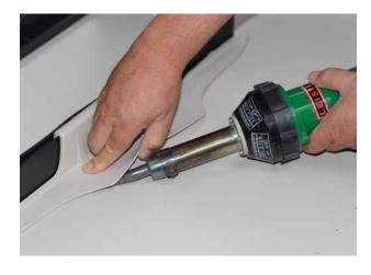
Temporary 2-point fixing of the Sika SolarClick sections along the inner end with a handheld hot-air welding gun.
