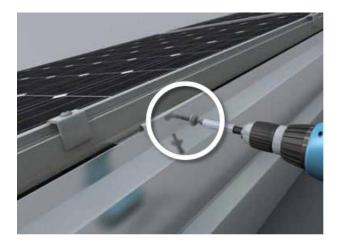
Fasten the wind deflectors in place using self-cutting thin sheet screws at each wind guide cap.
