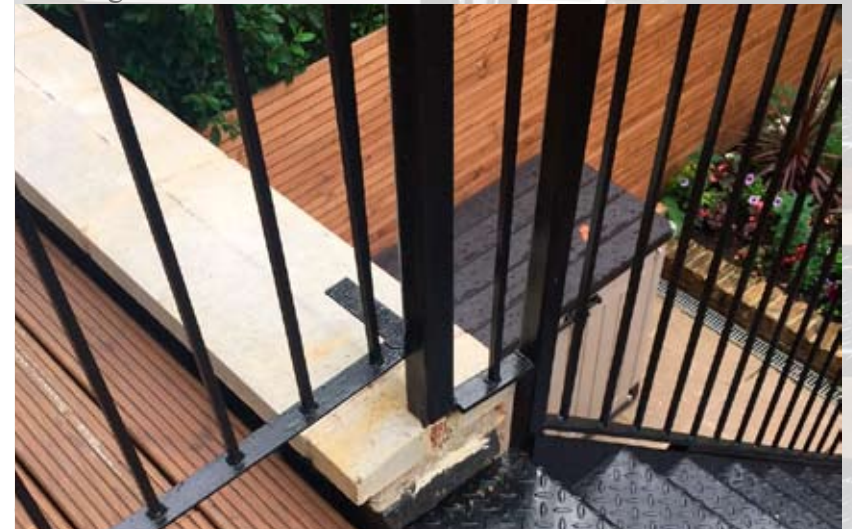
Existing intrusive Fence
