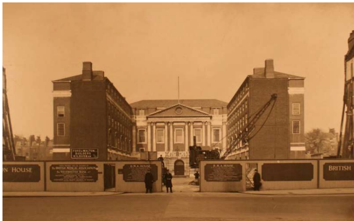
Early stages in the construction of Wontner Smith's extensions for BMA House in 1929.
