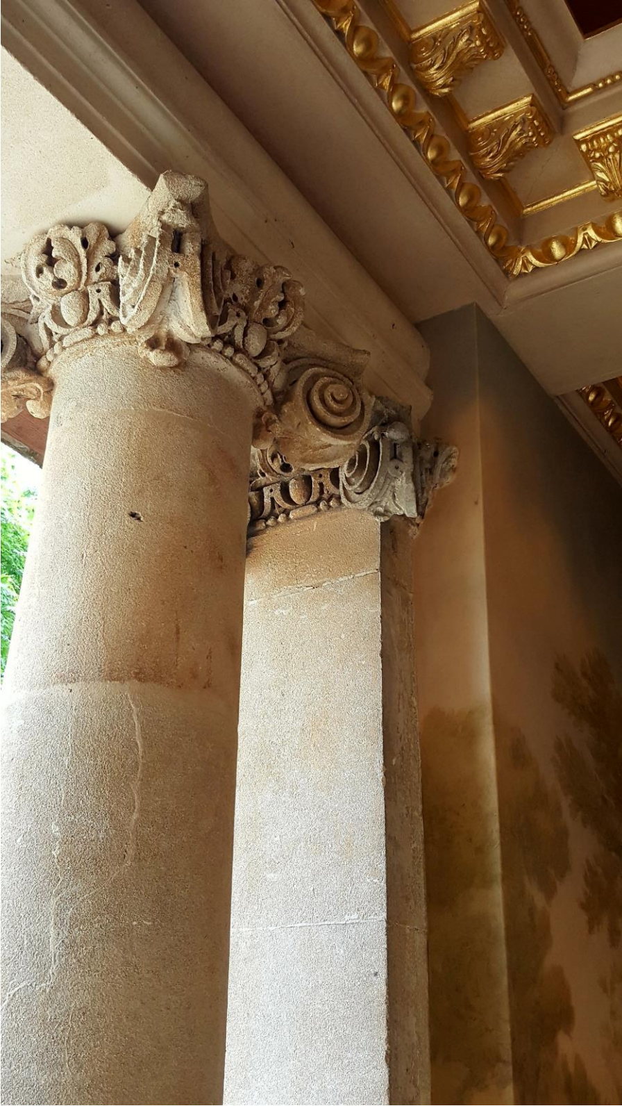
Fig 3. Pilaster/entablature head detail (June 2017)
