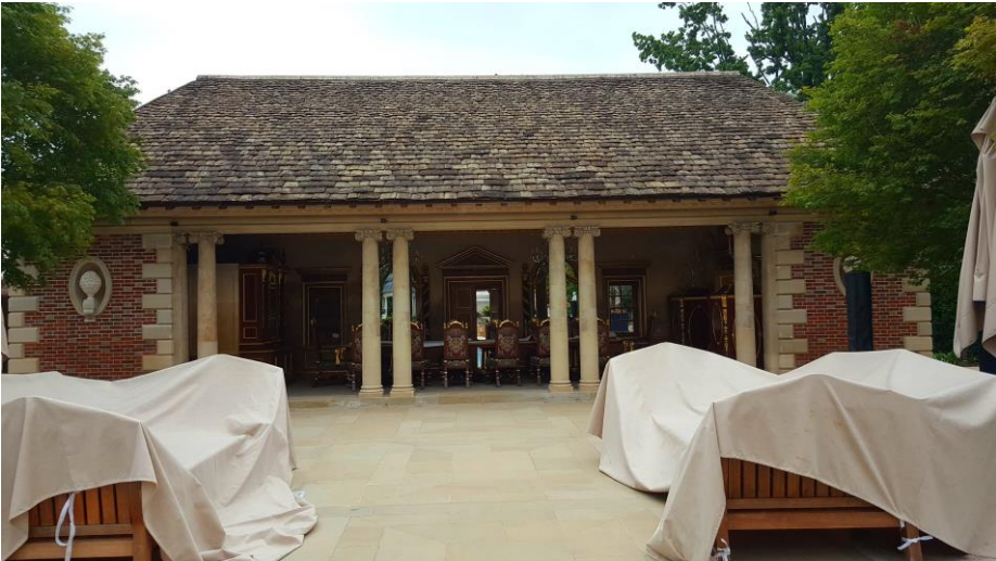
Fig 1. Peto Pavilion frontage from south-west (June 2017)
