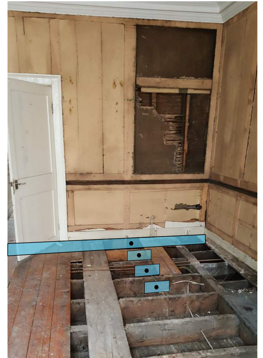
Figure 3, Spine Wall Strengthening Location
