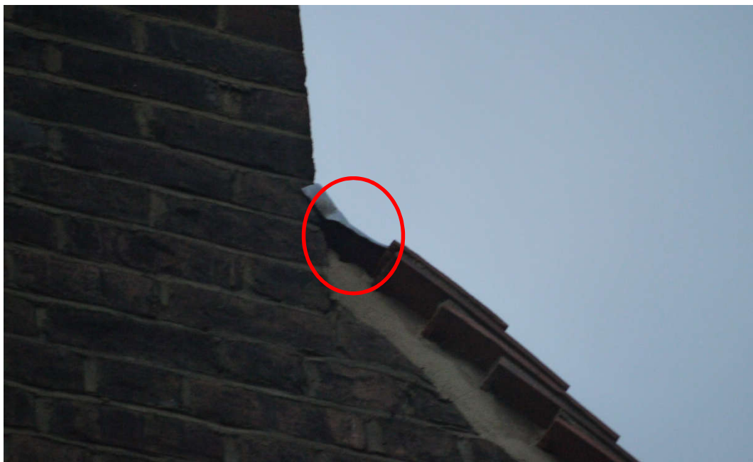
Figure 6. Close up of the gap under lifted flashing around the south-east chimney breast
