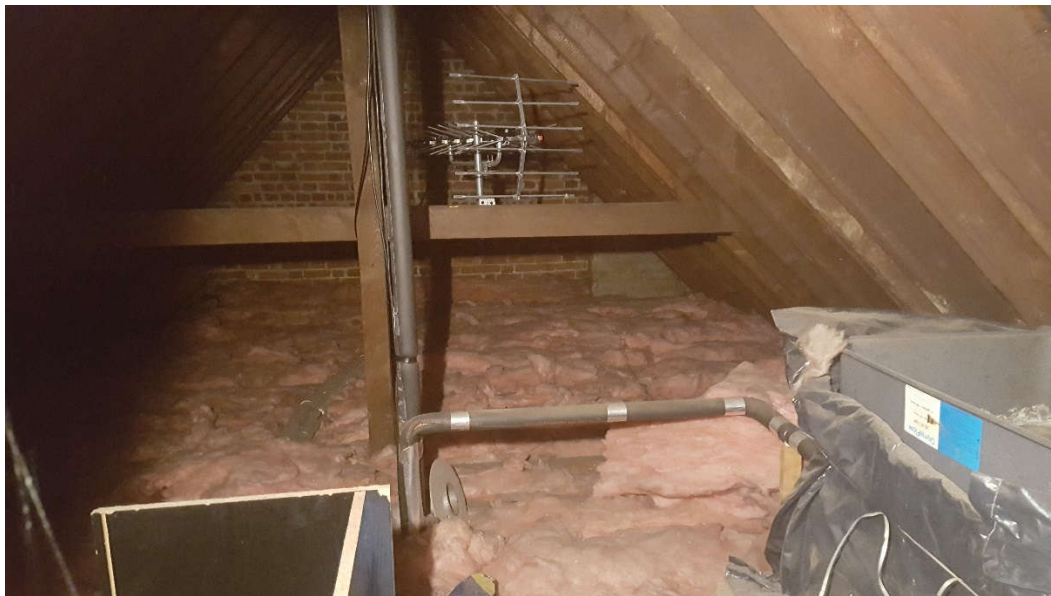
Figure 1. Inside the loft space during the internal inspection
