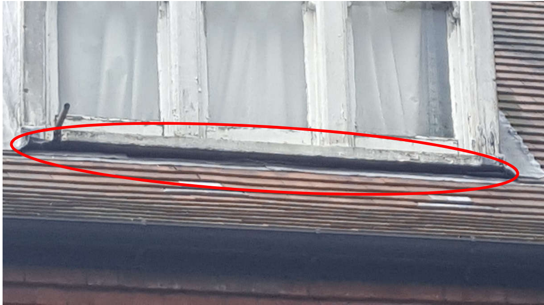
Figure 6. Close up of the gap under lifted flashing around the south-east chimney breast
