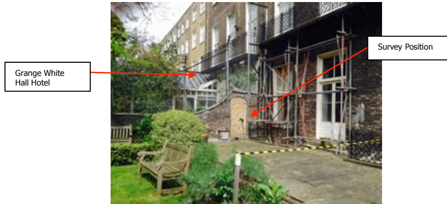
View of Survey Position (Looking north)
