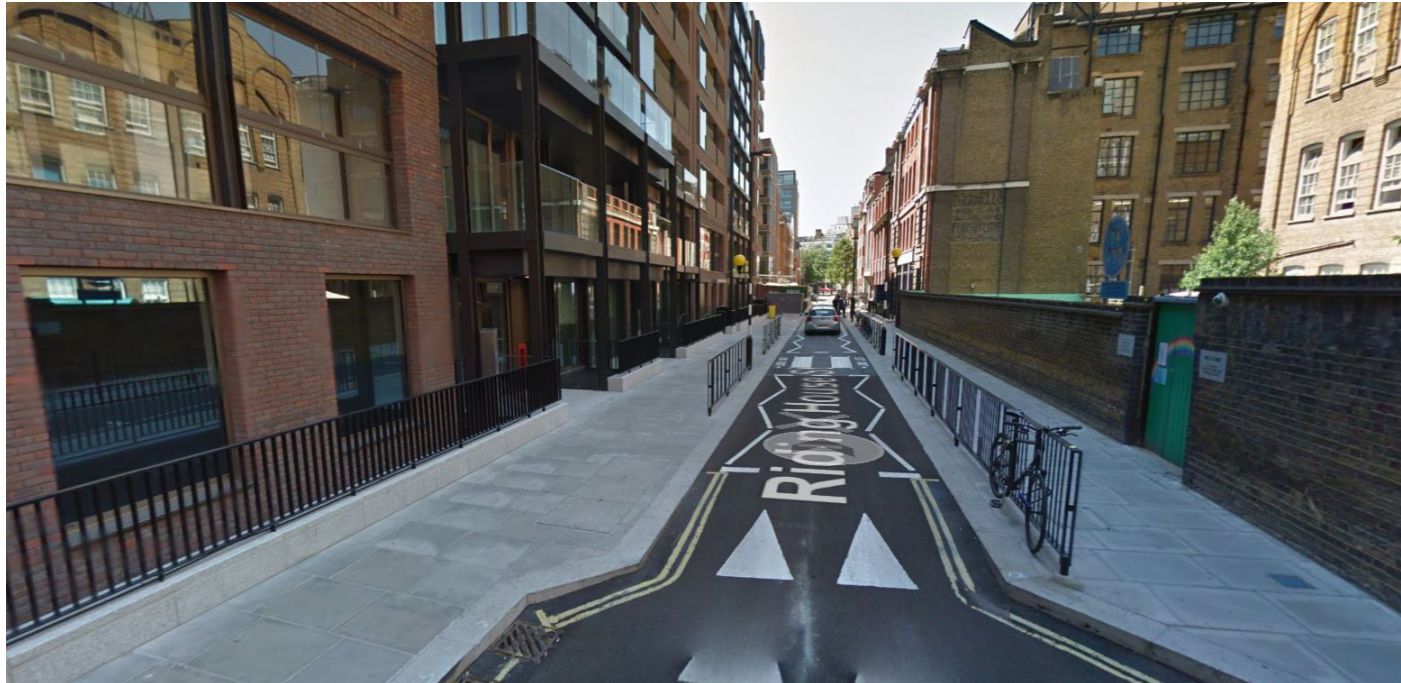
View south west along Riding House Street
