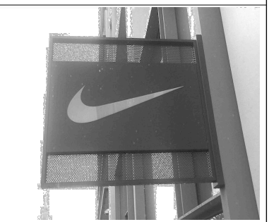
S8 SIGN REFERENCE IMAGE SIGN EXAMPLES SHOWN TO BE CONSTRUCTED WITH METAL MESH & SOLID STEEL SHEET PORTION ALLOW TO POWDER COAT ALL TO PREVENT RUSTING & CONCEAL ANY MANUFACTURER IMPERFECTIONS
