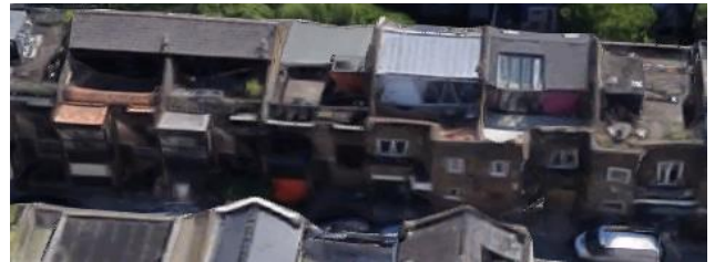
Figure 4. Assessed windows at 78-86 Camden Mews
