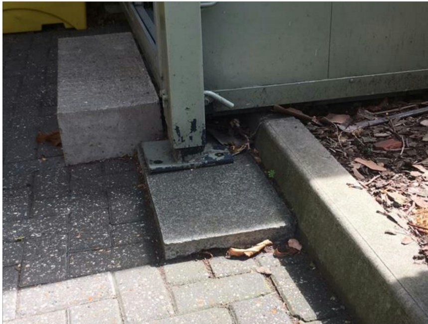
Fig. 3 Existing supports for the office building
