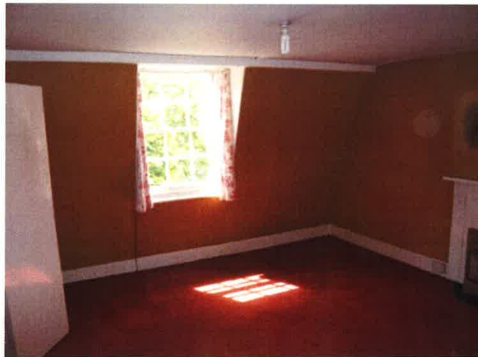
Overhaul and repair sash windows. Retain skirting and floorboards.
