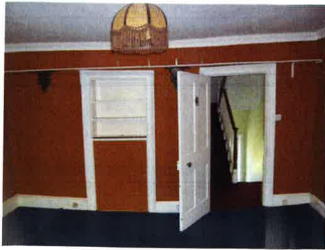
Existing alcove and shelving removed and opening reinstated with new door.
