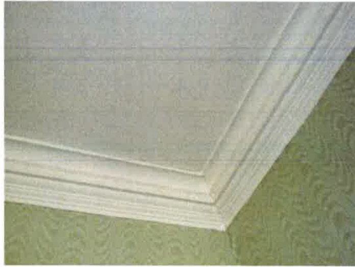
Existing ceiling and cornice to be retained and repaired.
