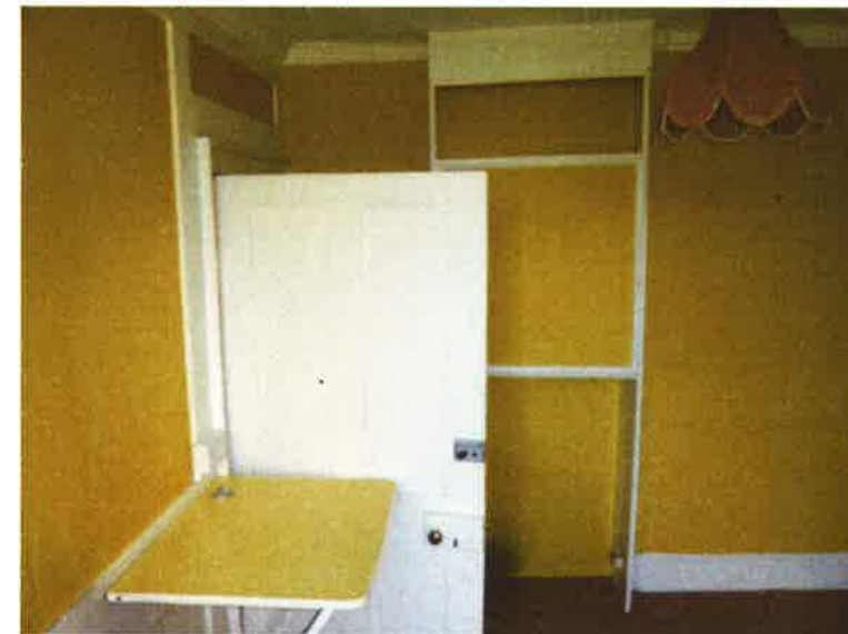
Strip and repaint timber door. Retain skirting and architrave. Retain and repair cornice.
