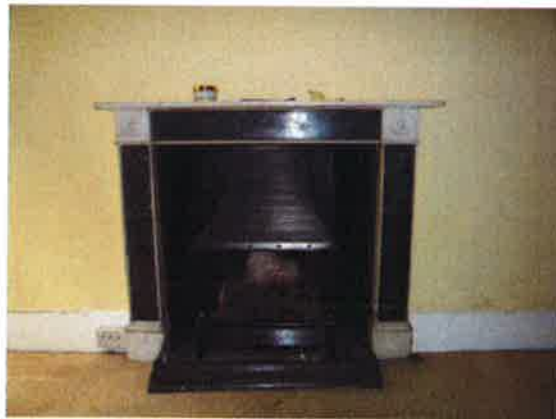
Retain fireplace surround and reinstate hearth.
