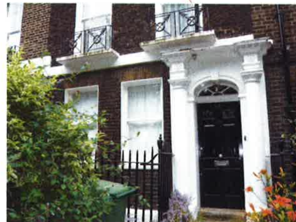
Retain & overhaul metal railings around existing lightwell, replace missing metal slim arrowhead to match existing. All external features are to be retained and overhauled
