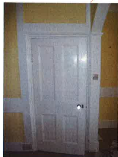
Strip and repaint all timber doors.
