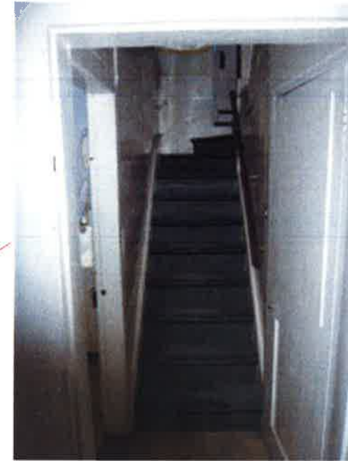
Strip and repair existing wooden staircase and balustrade.
