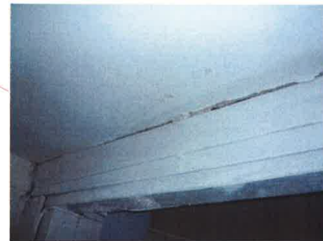
Retain and repair existing lath and plaster ceiling from above.
