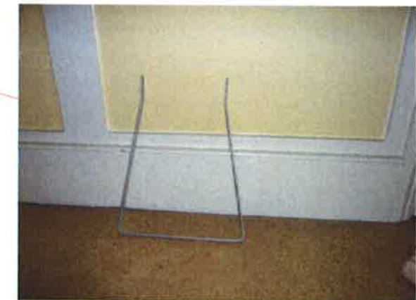
Retain, strip and paint skirting board.
