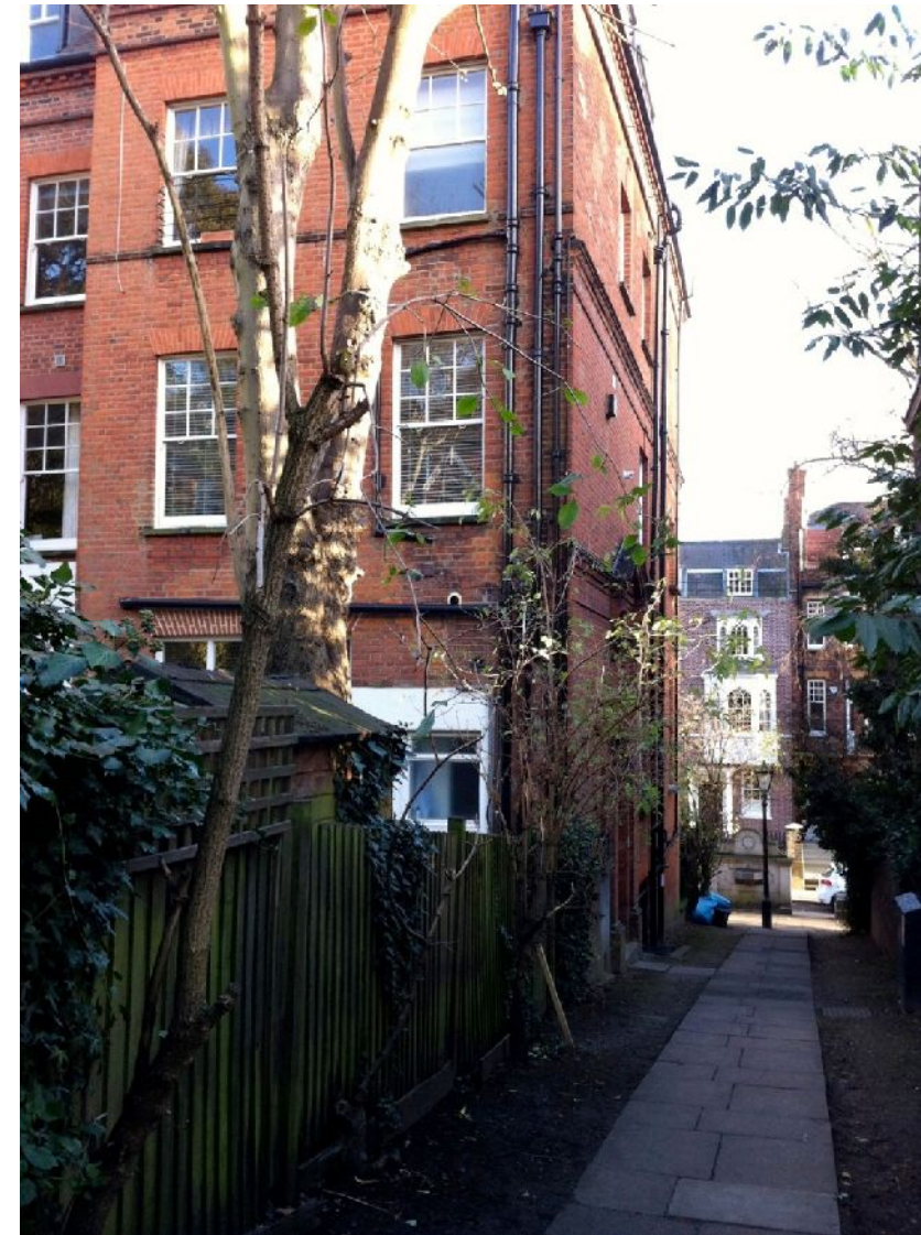
View of rear of property as existing from Well Walk Passage
