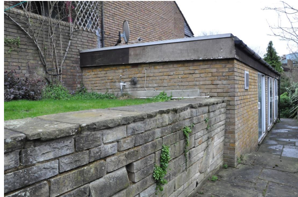
Existing swimming pool and passage along the boundary wall
