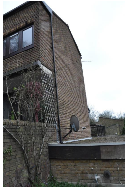
View to the South Western facade
