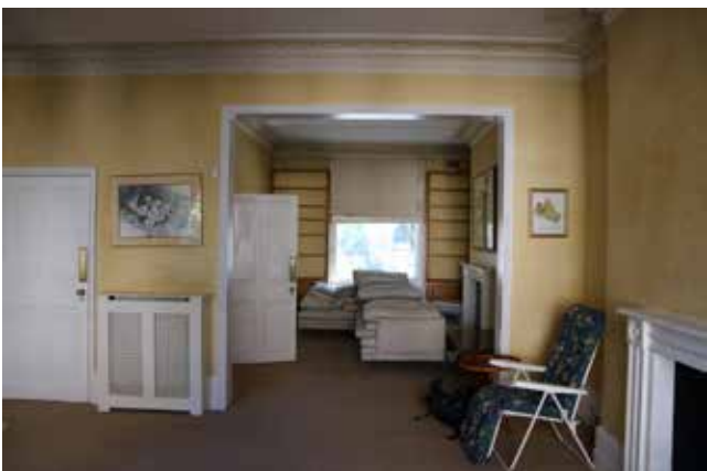
First floor front and rear rooms
