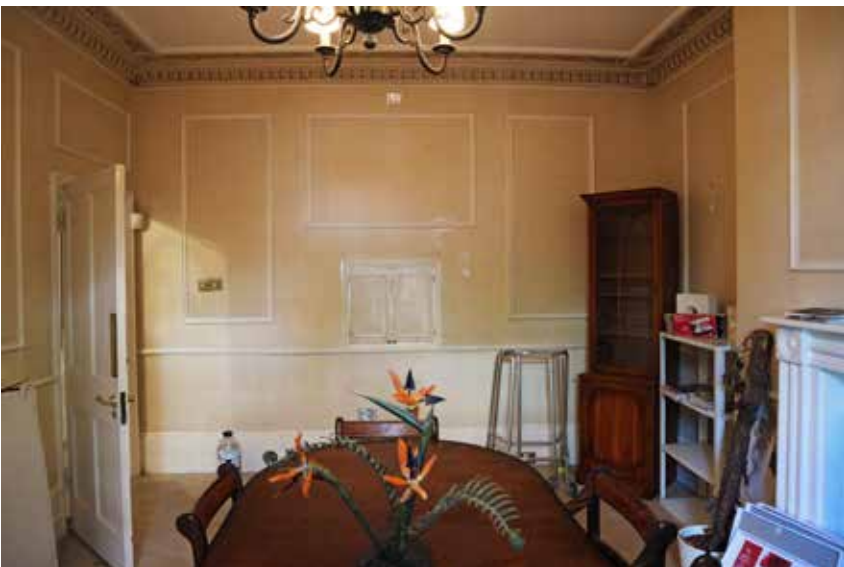
Ground floor front room spine wall
