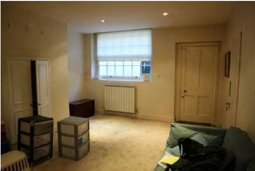
Basement front room
