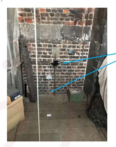
Cable rises through existing hole and connects into new adaptable box which replaces existing. Cables then are taken through he existing conduit to the upper levels.
