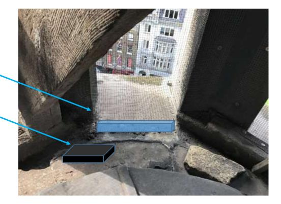
The protective mesh is not fixed well, therefore new galvanised channel sections are to be fixed at the base of the mesh using 2 resin fixings channel. The mesh can then be fixed into the channel by stainless steel self tapping screws. This will provide a longer term protective fixing method.
