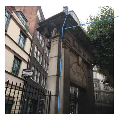
MICC cable to be dressed into contours of the stone archway and fixings to be within the mortar sections only. MICC cable to be painted with an exterior grade paint to a shadowed colour of the stone archway. Architect to approve colour selection prior to painting.
