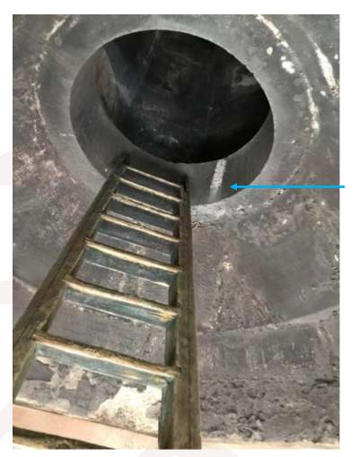
PVC coated rigid metal copex to be taken to a up to spire section. Copex to be cleated into mortar sections. Rigid copex type requires minimal fixings to be secured. Copex to be taken through existing opening. <u>No</u> additional hole is to be drilled for the cable.
