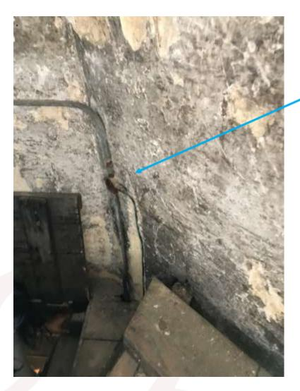
Cables to enter chamber via existing conduit. New adaptable box is to replace existing. Old luminaires and conduit to be removed. Cables to each clock face run horizontally between each of the 4 clock reveals. Cable clips to be fixed into Mortar and not stone.
