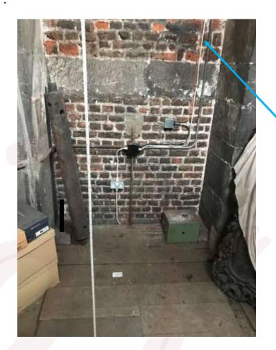
Cables to follow existing routes. Old cables to be removed. Cables to rise from new adaptable box in loft chamber and out through existing hole to parapets.
