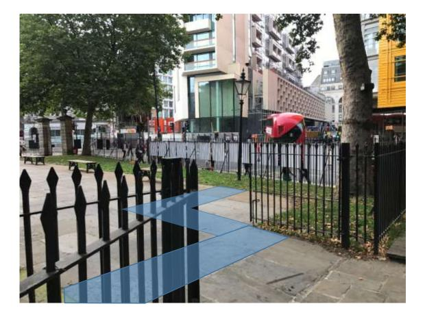
Cable taken under marked slabs and laid in a hand dug trench (500mm minimum depth) to post location.
