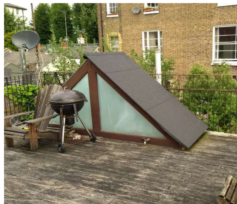
Site Photograph 3 - 8 Albert Terrace Mews Roof Terrace & Existing Access Hatch
