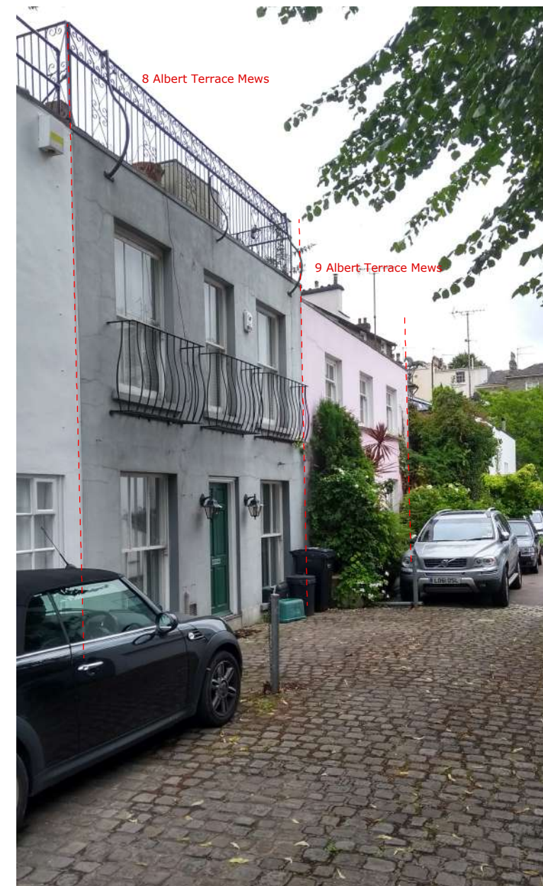
Site Photograph 2 - 8 Albert Terrace Mews looking East
