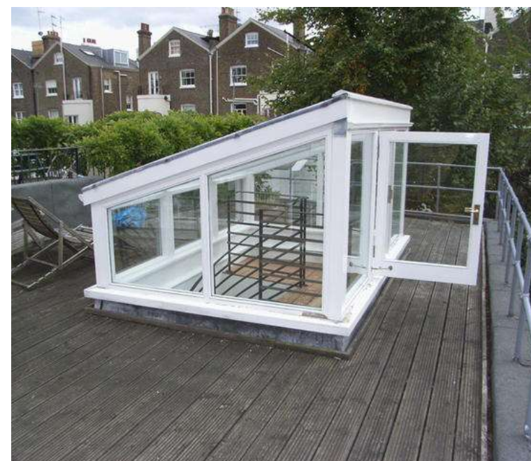
Site Photograph 4 - 7 Albert Terrace Mews Roof Terrace & Access Hatch
