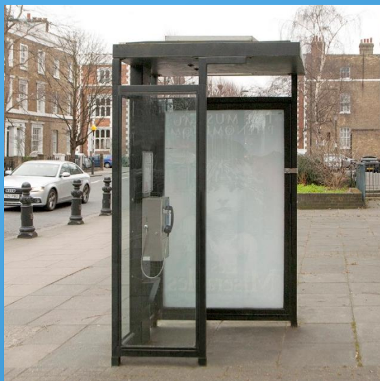
Left Side of the kiosk showing the rear of the existing advertisement display
