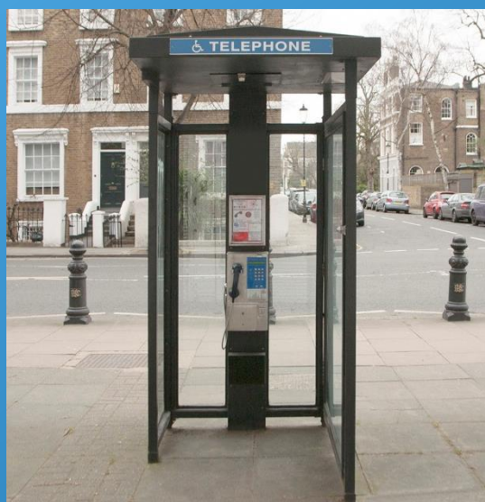
Front of the kiosk as seen from the pavement side showing open covered kiosk and accessible payphone
