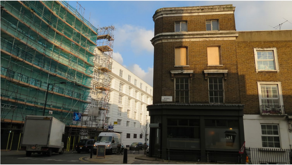
Fig 8 View showing existing Crittall type window on the third floor
