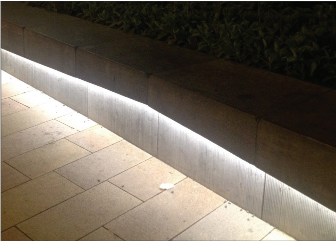
Integral lighting strips to the raised planters
