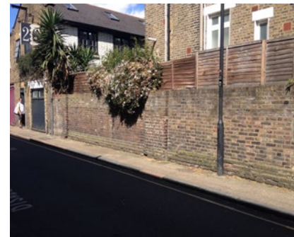
BUILDING AT THE REAR
