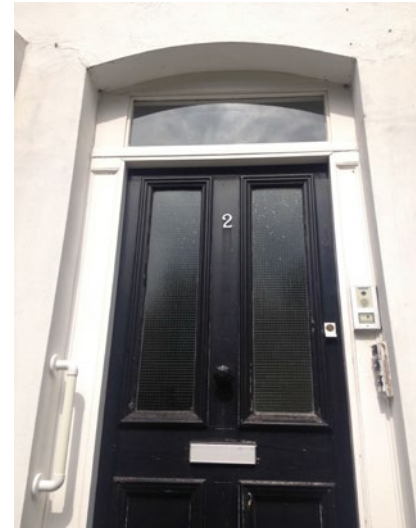
MAIN HOUSE FRONT DOOR
