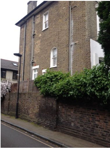
FLANK WALL OF 2 CAVERSHAM RD
