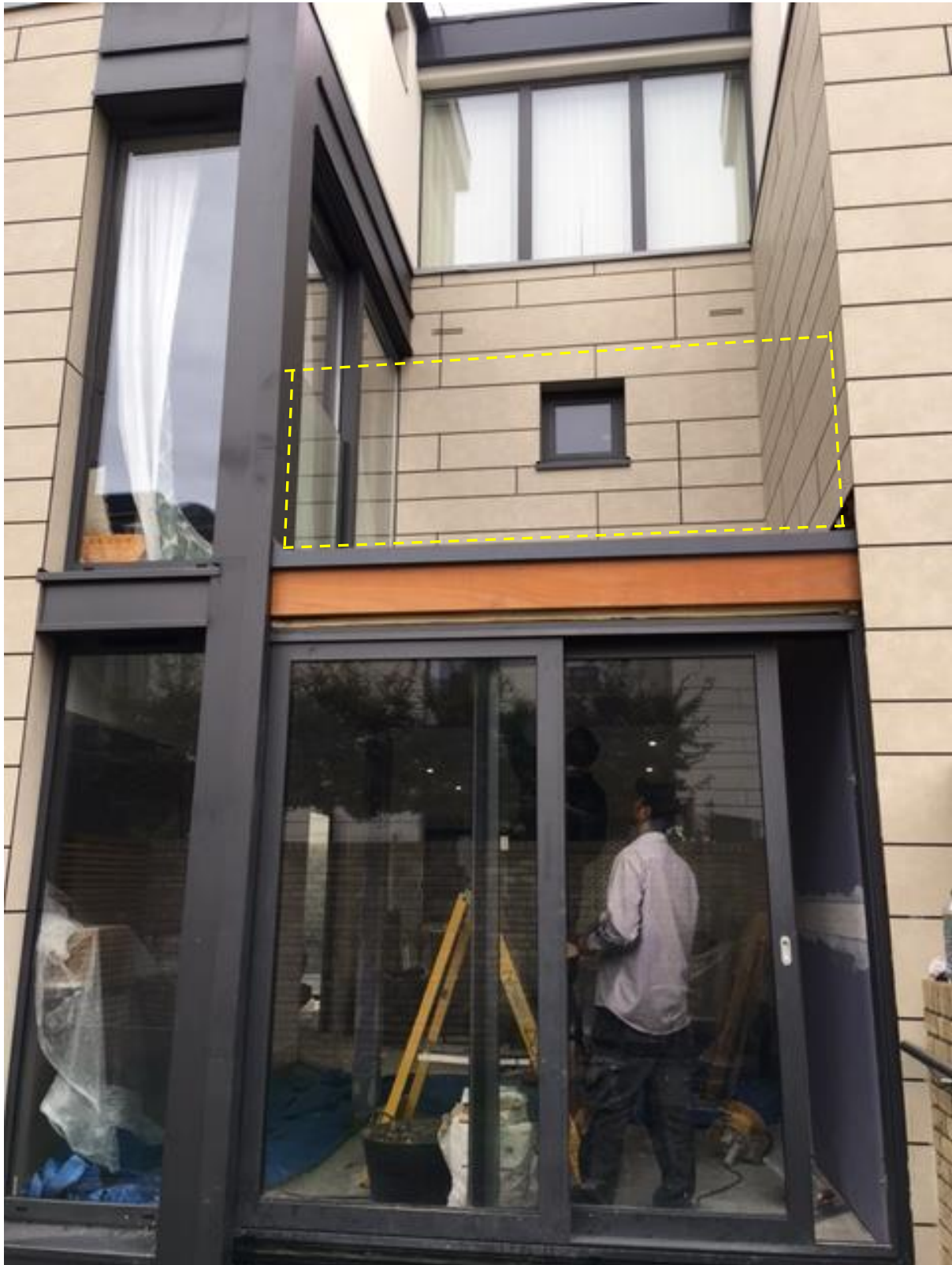
Photo.1 View back towards No.10 indicating position of glazed balcony.
