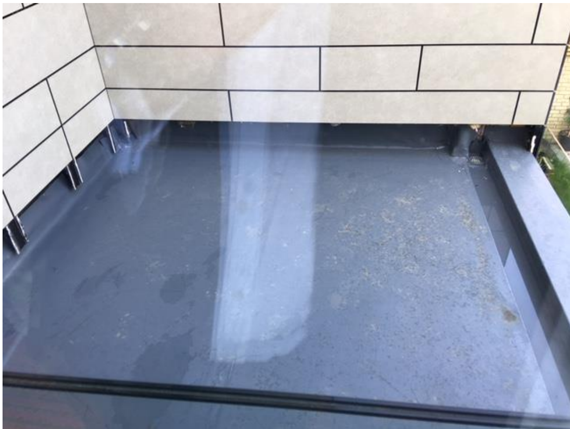
Photo.3 New roof in place for balcony
