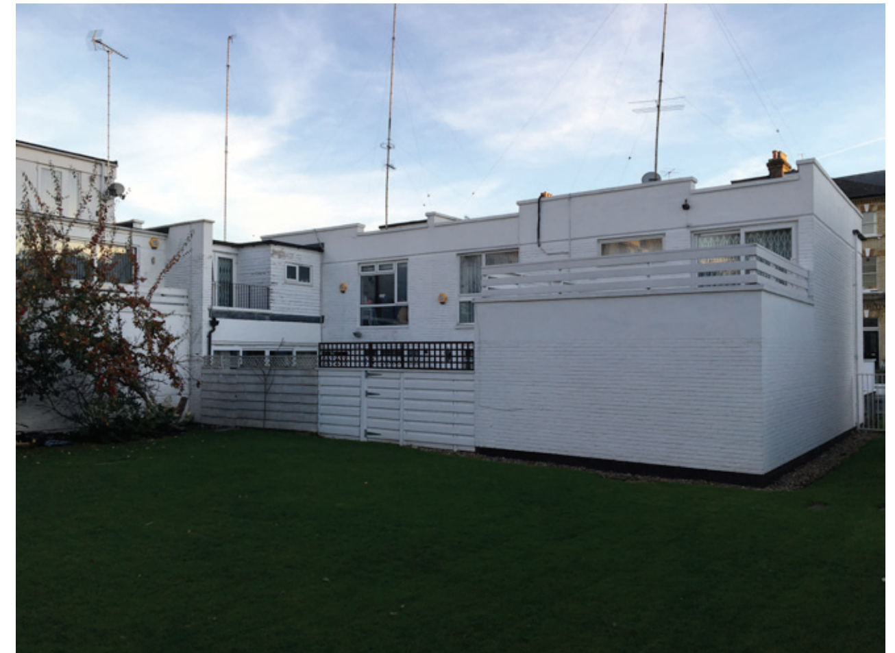
View of rear of 106 King Henry's Road from communal garden
