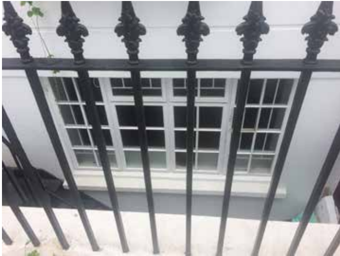
6 Mornington Terrace - view into basement window
