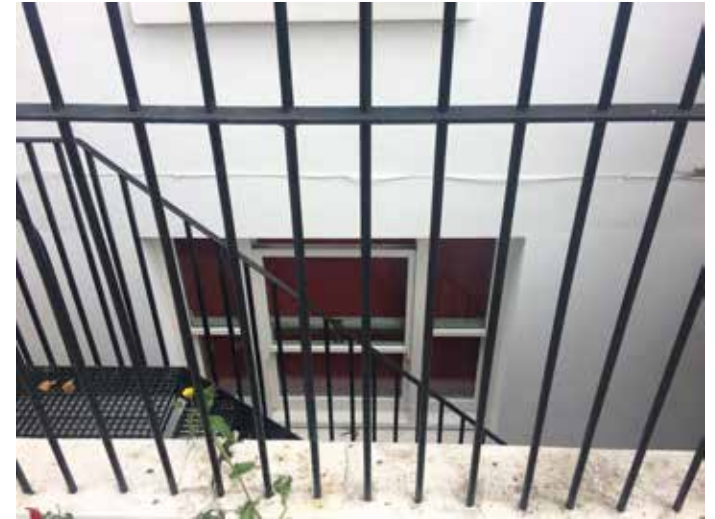
4 Mornington Terrace - view into basement window
