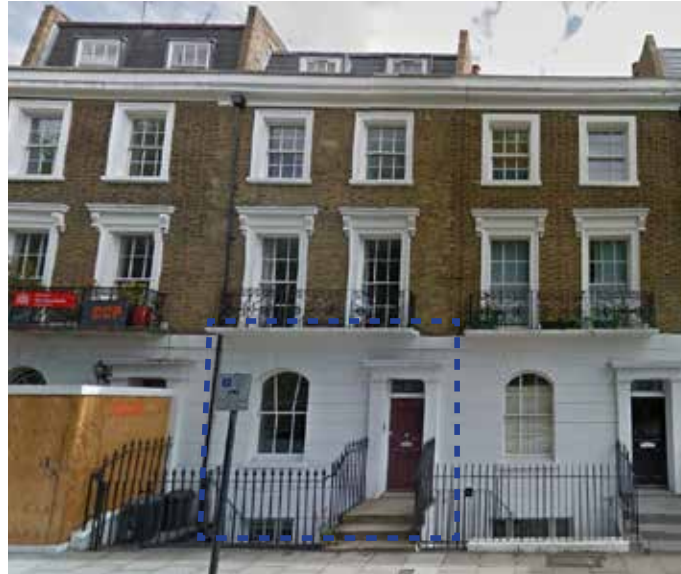
5A Mornington Terrace and adjoining neighbours
