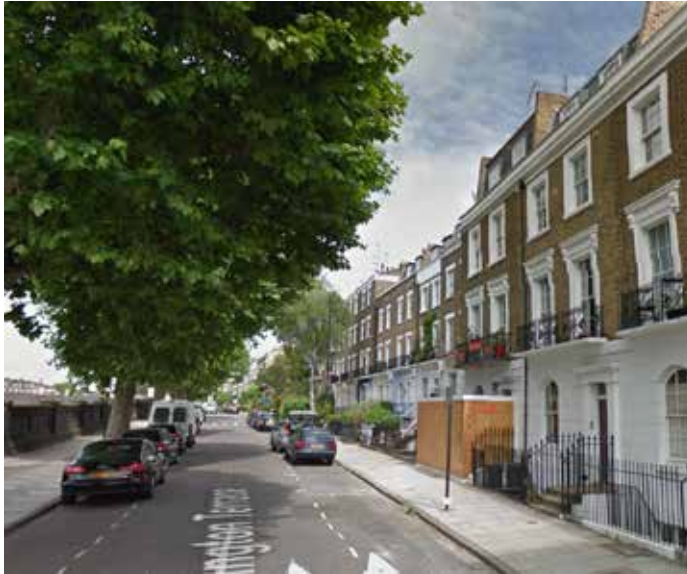
Street view showing relationship to railway cuttings
