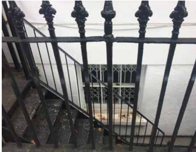
Existing window, 5A Mornington Terrace
