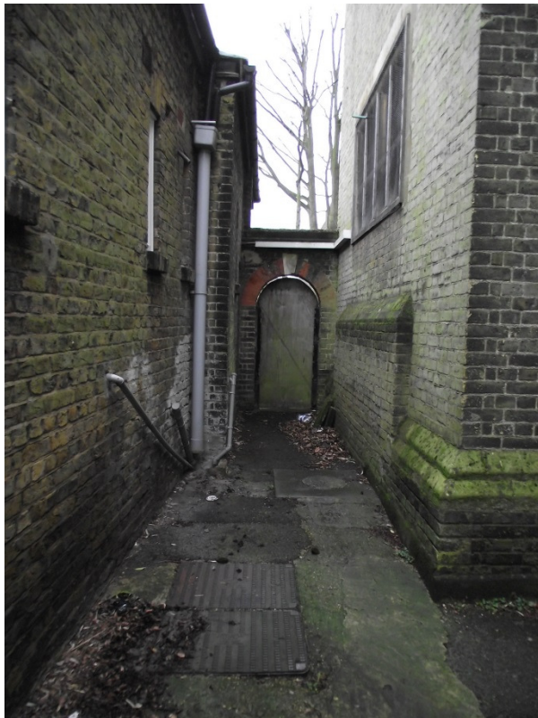
Passageway with existing gate
