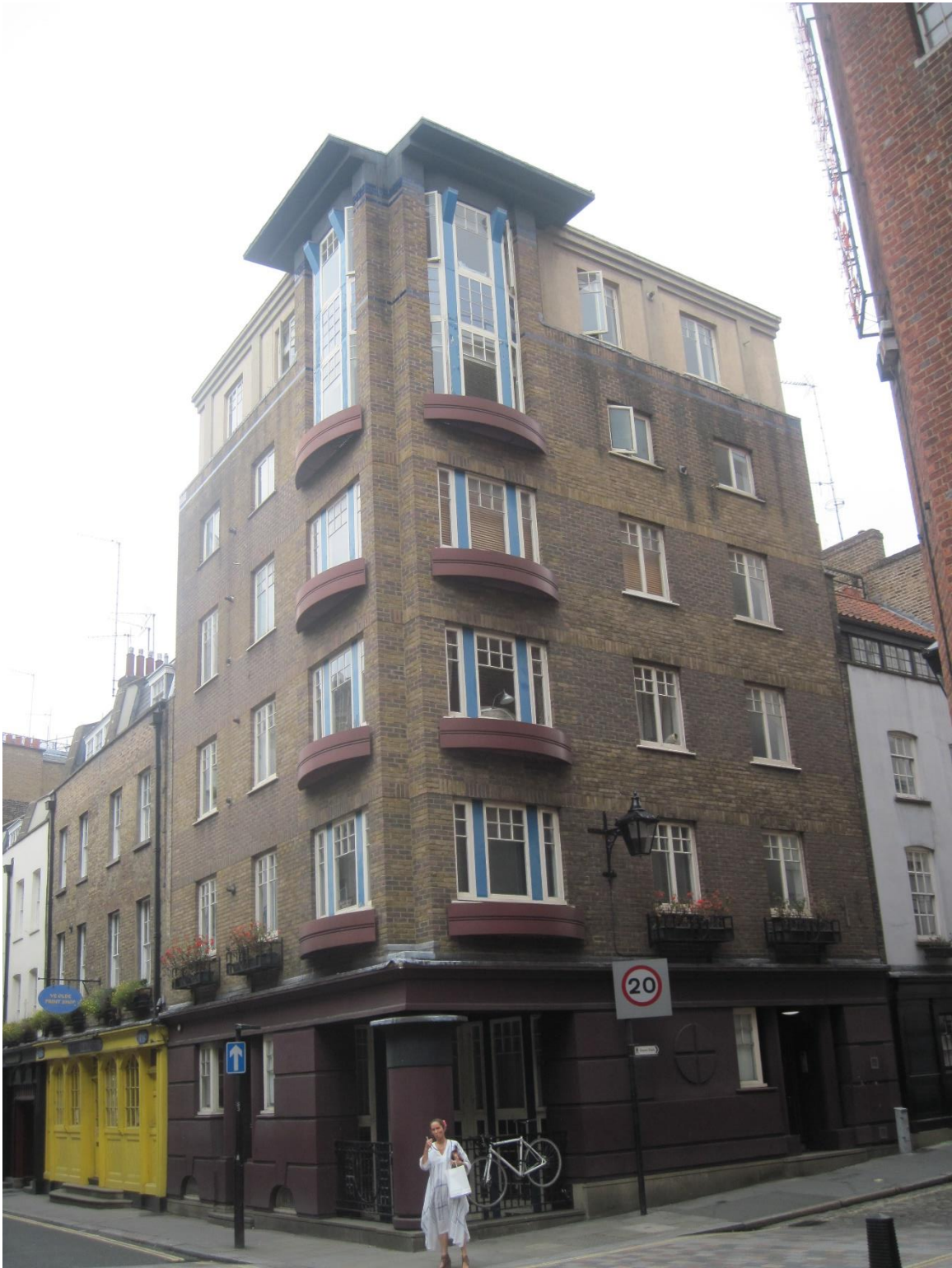
Photograph No.1 - 19 Mercer Street seen at the junction with Shelton Street
