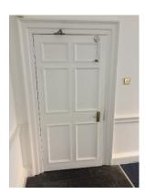
• **External Front door**: External door to building frontage to be retained and redecorated with white paint internally. Ironmongery retained. New access controls mounted to wall externally beside door.
