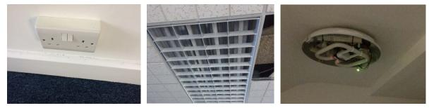
• **Ceilings:** All cornices to be retained and redecorated with white paint. The modern suspended grid ceiling to be strip out and replace with new plasterboard ceiling.
