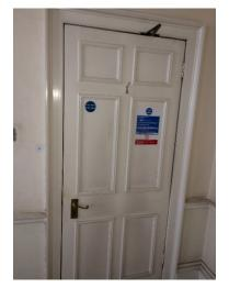
• External Front door: External door to building frontage to be retained and redecorated with white paint internally. Ironmongery retained. New access controls mounted to wall externally beside door
