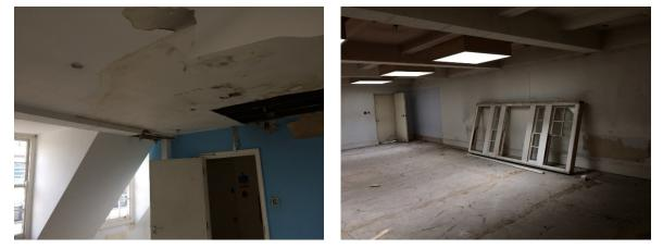
• Internal Walls: All existing walls and mouldings to be retained and redecorate with white paint; all exposed brick work walls to be covered with plasterboard decorated with white paint
