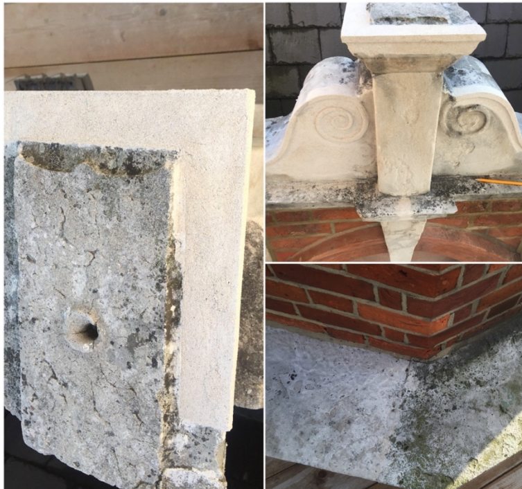
Detailed masonry works and doff steam clean to stone. Marked improvement lifting aged dirt from stone.
