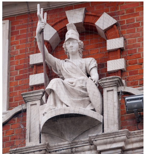
Detailed masonry works and doff steam clean to stone. Marked improvement lifting aged dirt from stone.
