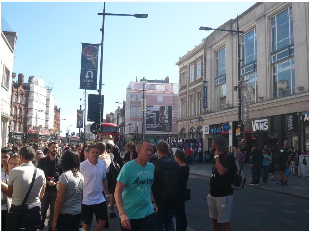
187 Camden High Street during sponsored restoration. Full working scaffold shrouded in 1:1 visual representation of host building with inset commercial area in the Camden Town Conservation Area.
