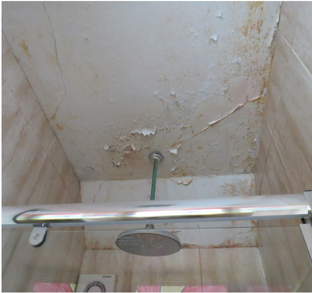
fig 6 & 7. 98 Highgate West Hill - internal and external damp
