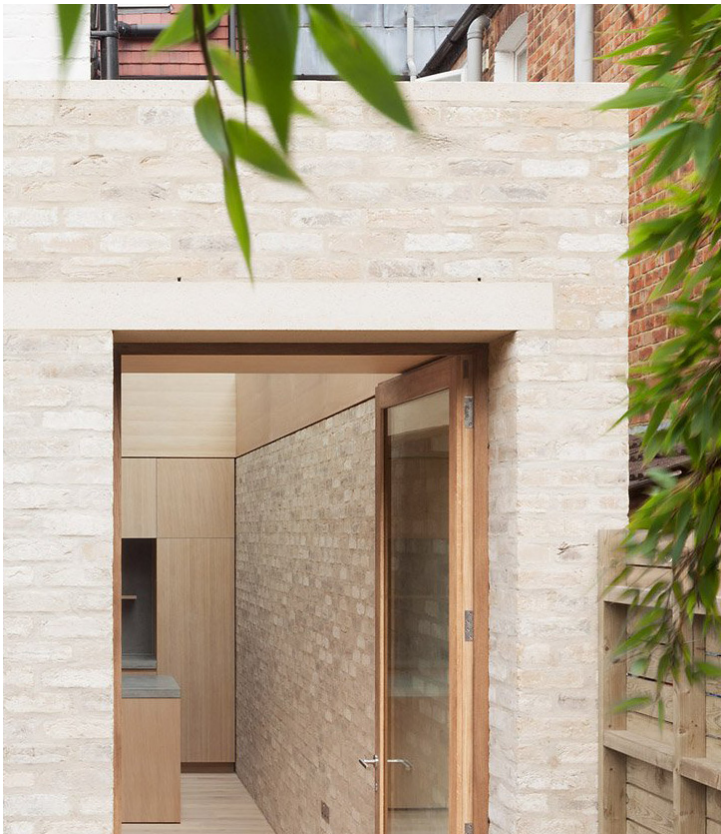
Reference for of lime slurry finish into a facing brick wall.
