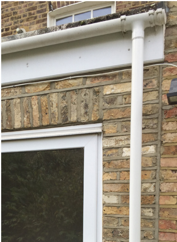
Mismatched pointing colour into back elevation.
