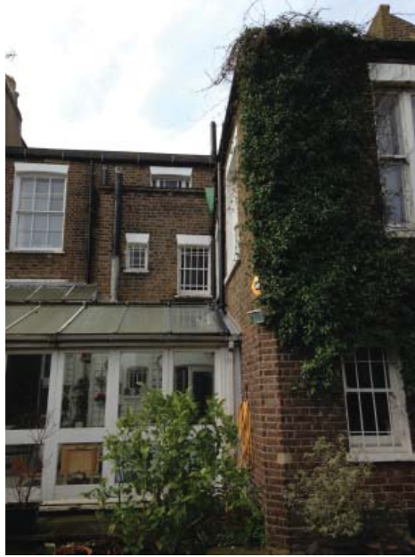
Photo 02: Rear facade, house 4 Boscastle Road (photo March 2017)
