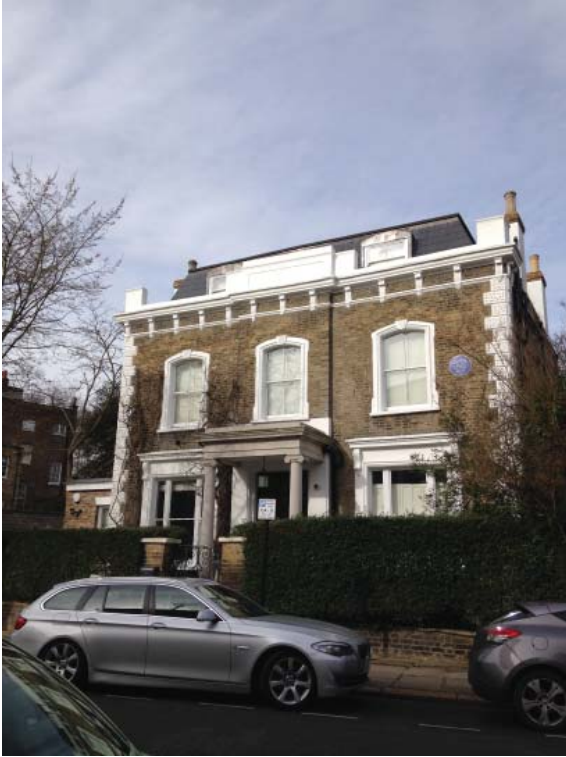
Photo 04: Example of similar roof loft conversion, on Dartmouth Park Road. (photo March 2016)
