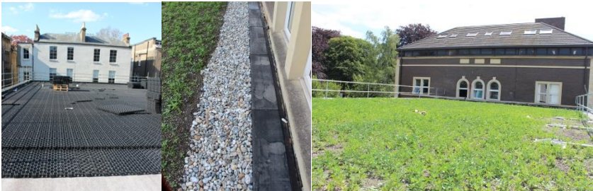
University of Bristol void former installation and completed blue / green roof
