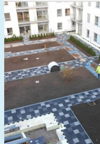
A work in progress view of a similar roofscape where attenuation has been blended with increased amenity value
