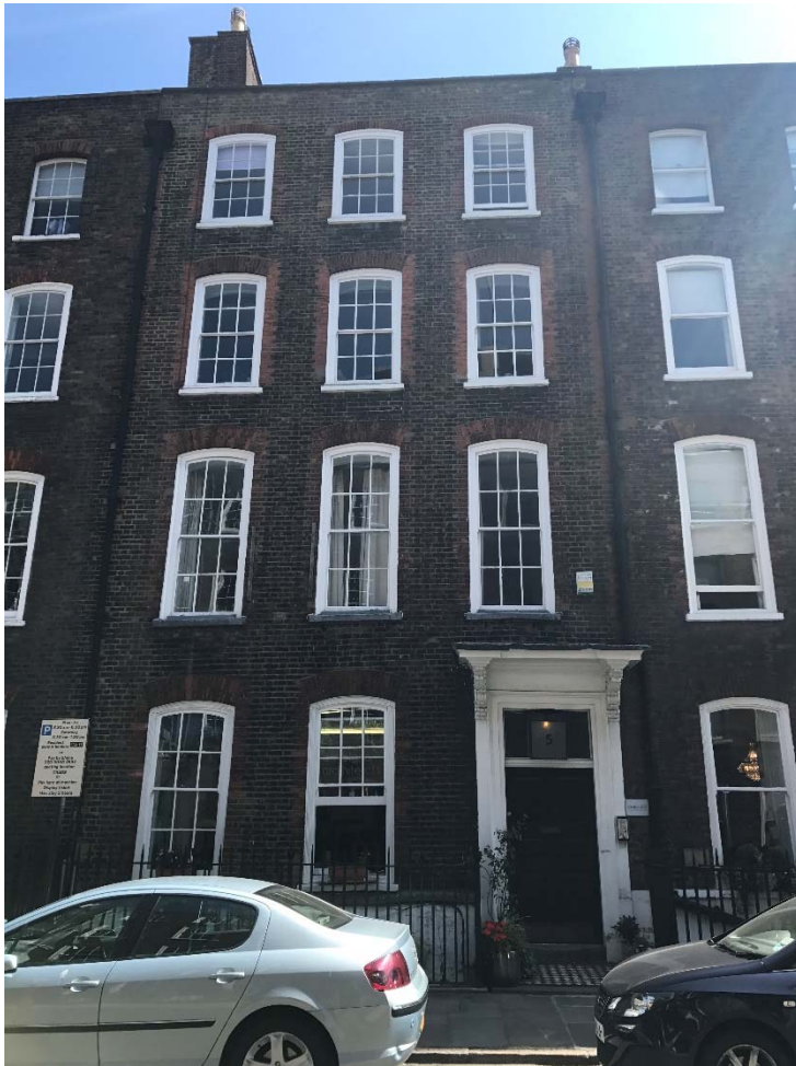
Fig 1 Street View: 5 Great James Street
