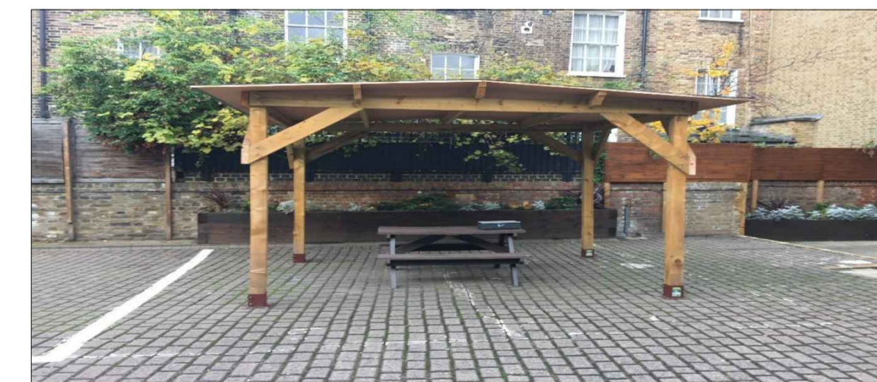
E - PICNIC STRUCTURE IS 3.0M X 2.5M, TIMBER CONSTRUCTION WITH FELT COVER ON ROOF
