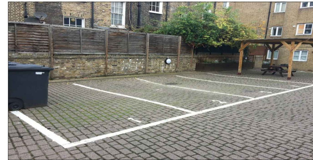
D - PARKING BAYS ARE PAINTED ON BLOCK PAVING, THERE ARE NO PARKING SIGNS IN OTHER PLACES
