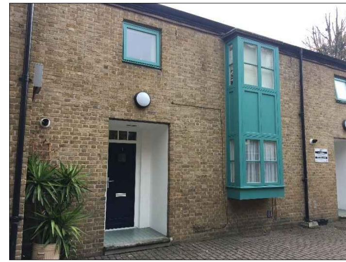
A - CCTV CAMERAS REMOVED FROM NUMBER 1 & 4 GREEN YARD
