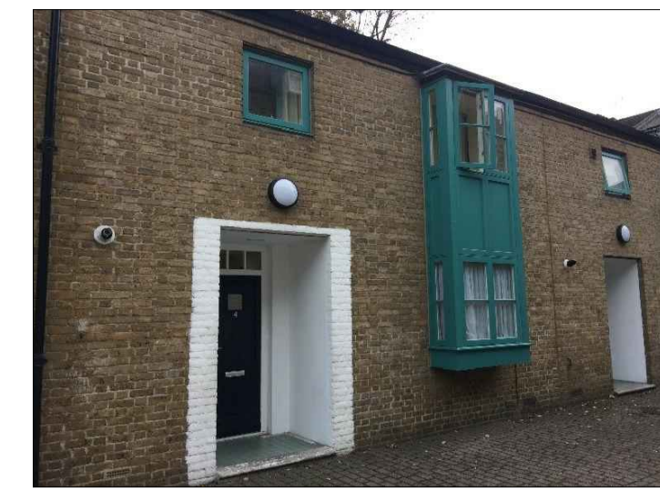
B - CCTV CAMERAS REMOVED FROM NUMBER 1 & 4 GREEN YARD
