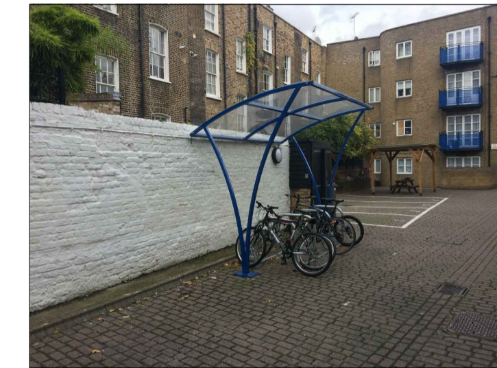
F - PAINTED WALLS FACE ORIGINS PROPERTY, BIKE SHED IS PRE-FABRICATED AND BOLTED IN SITU - PAINT TO WALL TO BE REMOVED IN ACCORDANCE WITH METHOD STATEMENT PLEASE REFER TO DESIGN & ACCESS STATEMENT. CYCLE STORAGE TO BE REPLACED WITH 2NO. FALCO CREA CYCLE STORAGE UNITS. LIGHTING TO LISTED PAINTED WALL TO BE REPLACED WITH HALF COACH LANTERN.
