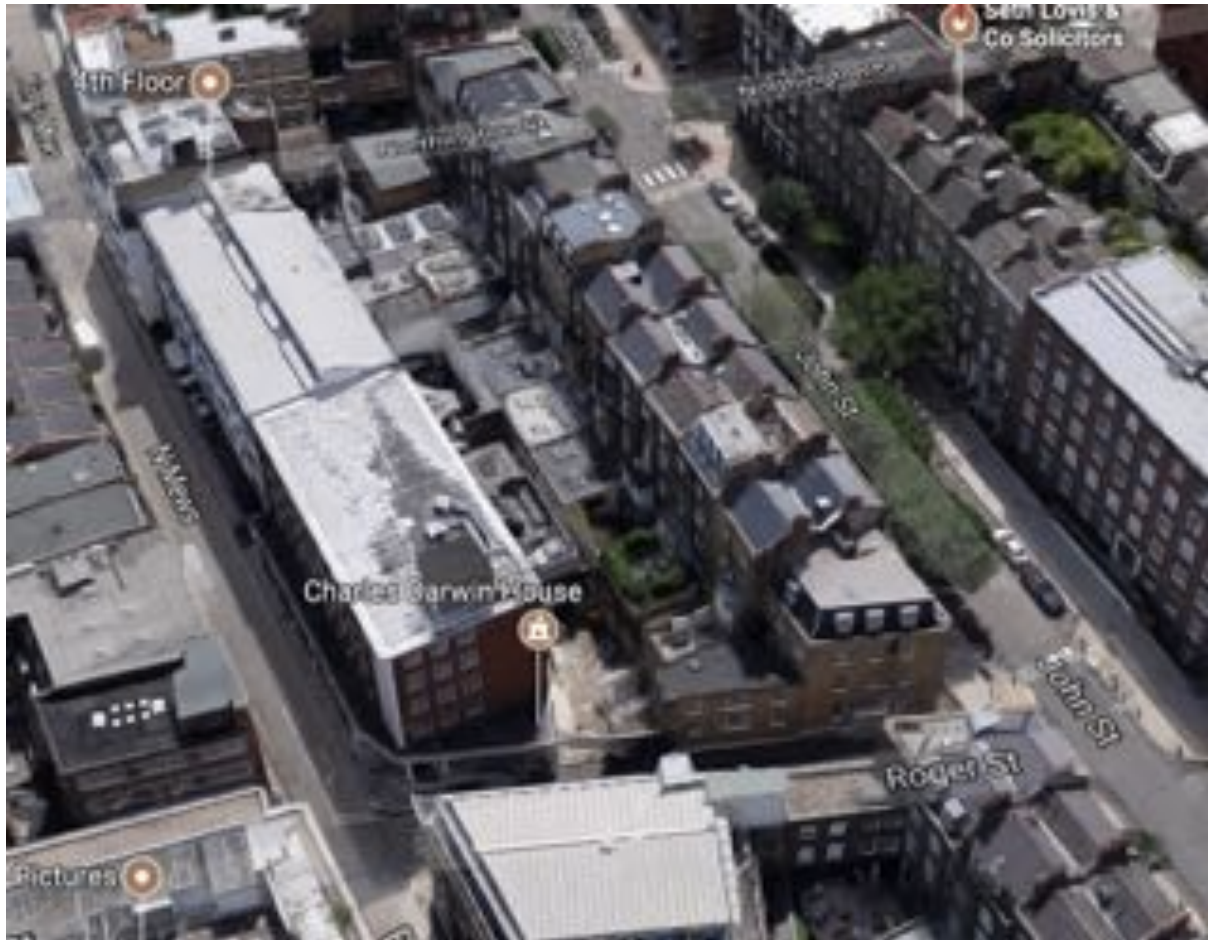
Image extracted from Google maps (for information only) showing the infill extensions to the rear of buildings along this section of John Street.
