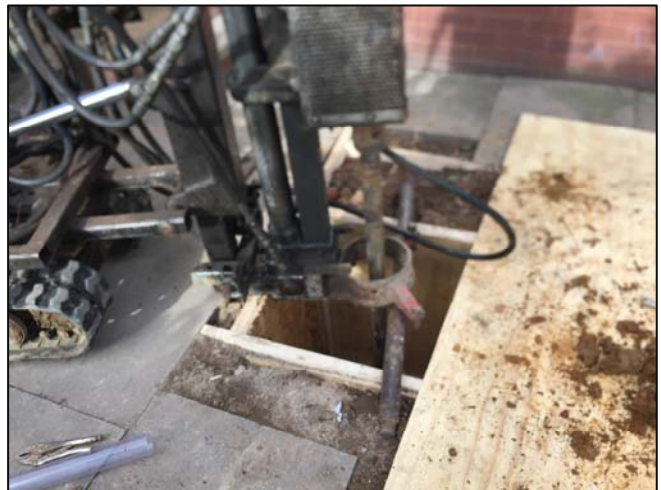
Location and view of WS1 and TP1 through patio with use of supporting boards
