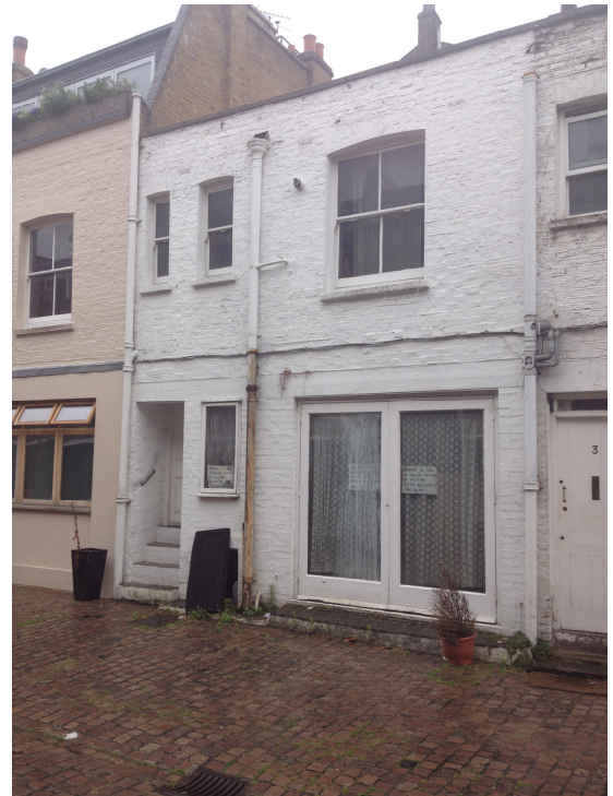
Existing view of the front elevation 2
