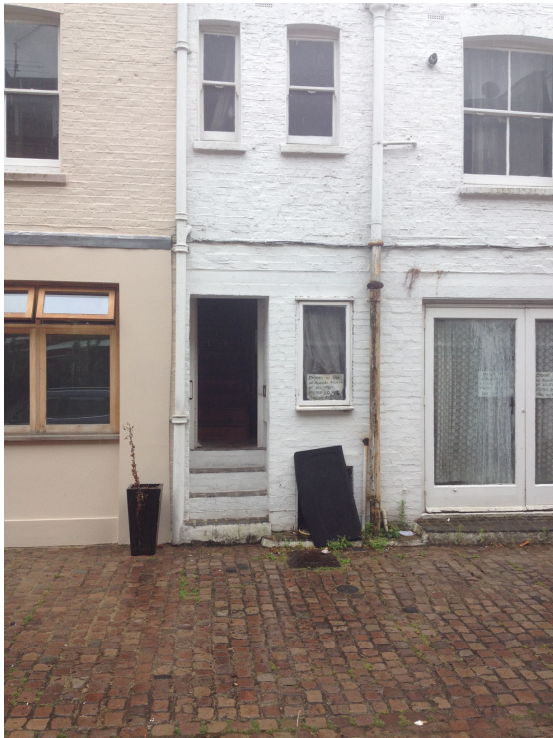
Existing view of the front elevation 1
