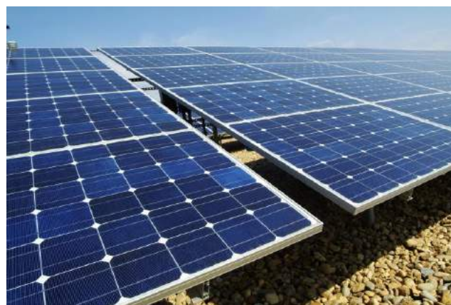
Figure 9: Monocrystalline PV arrays
