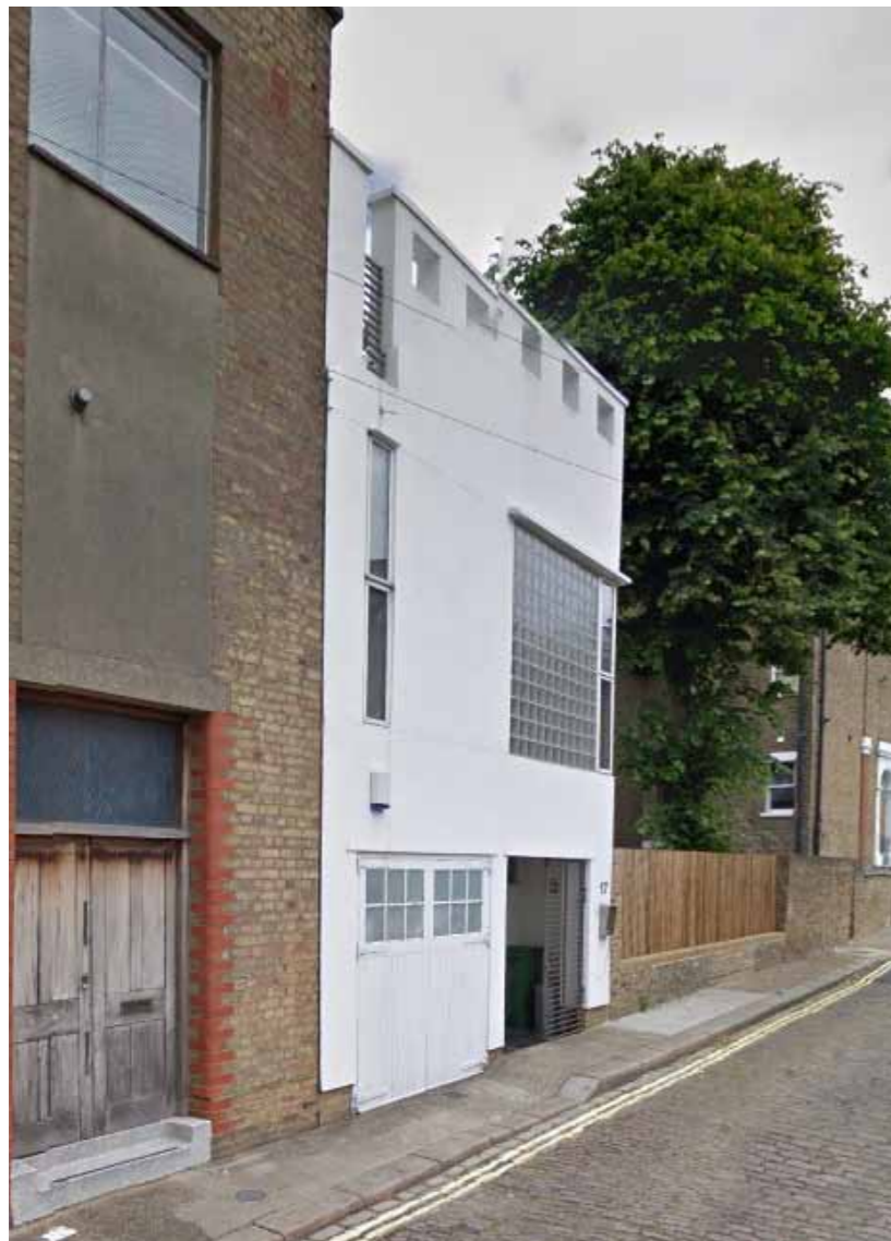
▲ View from the Mews (West)
