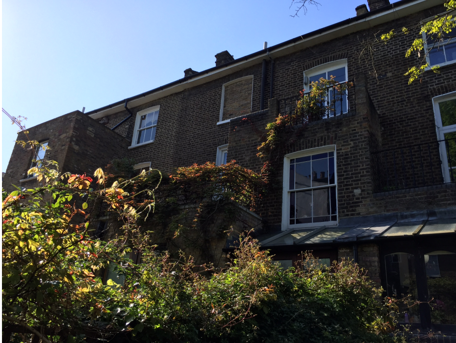
Rear of 21 Lawford Road – showing differing rear extension
