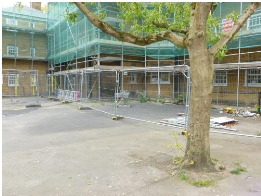
Existing central courtyard to be re-paved. Existing trees to be retained.
