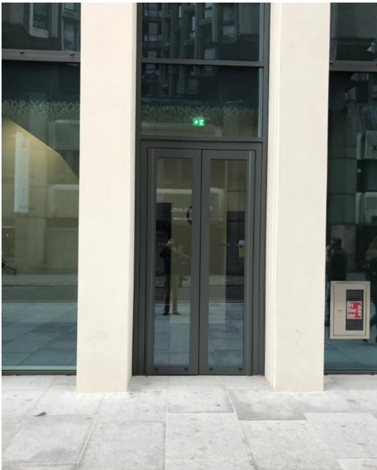
Existing fire exist door from adjacent offices.
