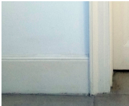
Fig 4: Architrave on Second Floor
