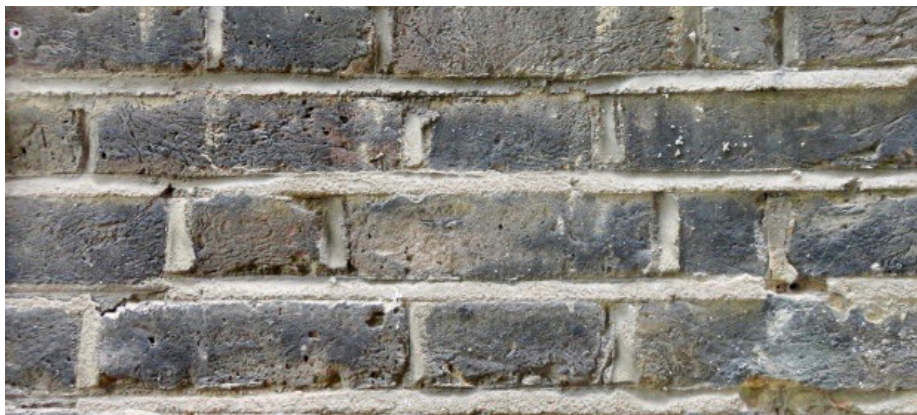
Fig 1: Existing Brickwork on Rear Facade
