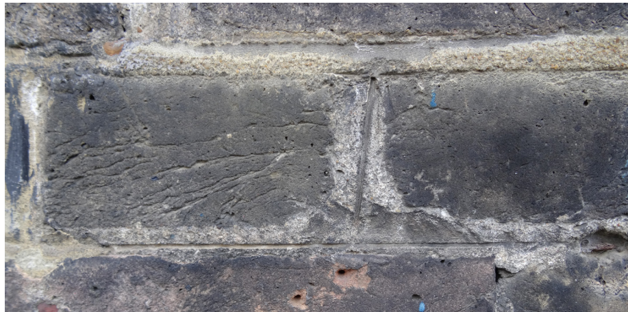
Fig 2: Existing Brickwork on Rear Facade
