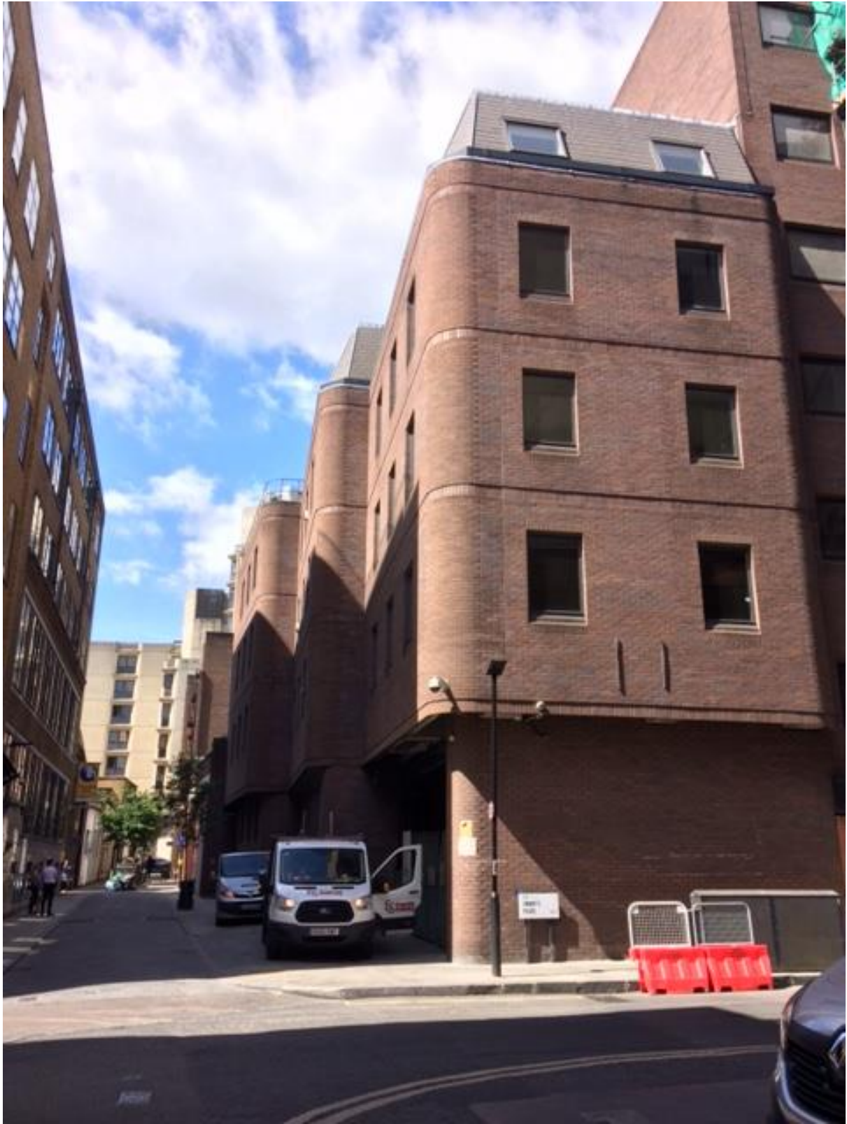
Photo 1 East Elevation – from Stukeley Street
